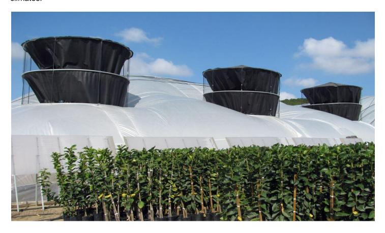
Our wind-assisted air-supported greenhouse structures are designed to be inherently organic, by preventing the entry of pest insects and by maintaining proper airflow to control humidity levels and reduce fungal pressures. Our greenhouse structures have been certified by the USDA for protection of crops against insects that vector disease, such as the Asian citrus pysllid, which carries Huanglongbing and has devastated citrus trees around the world.
